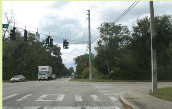
Curb ramps are missing along the north side of Plymouth Avenue at the intersection with Amelia Avenue.
